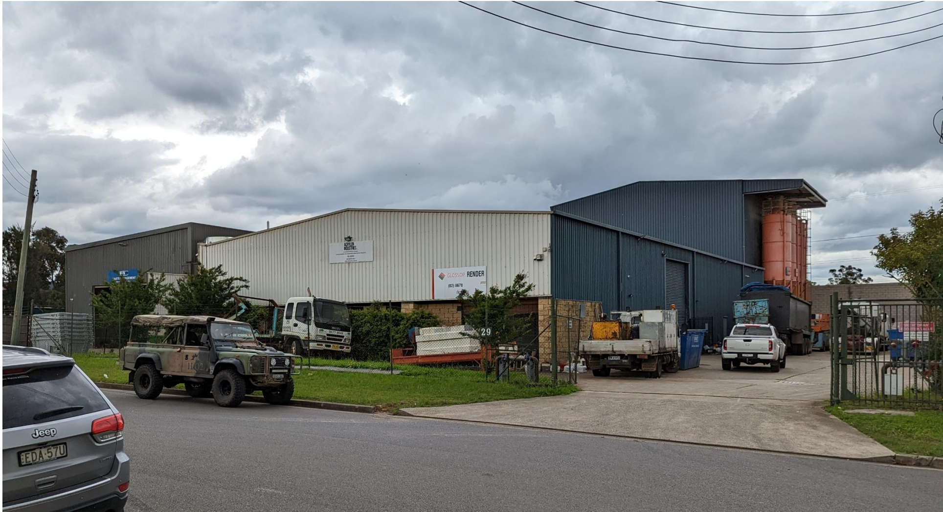
Figure 13.2. View of the front of 29-31 Plasser Crescent (Lot 15 DP 263353) showing dominant Site features.
