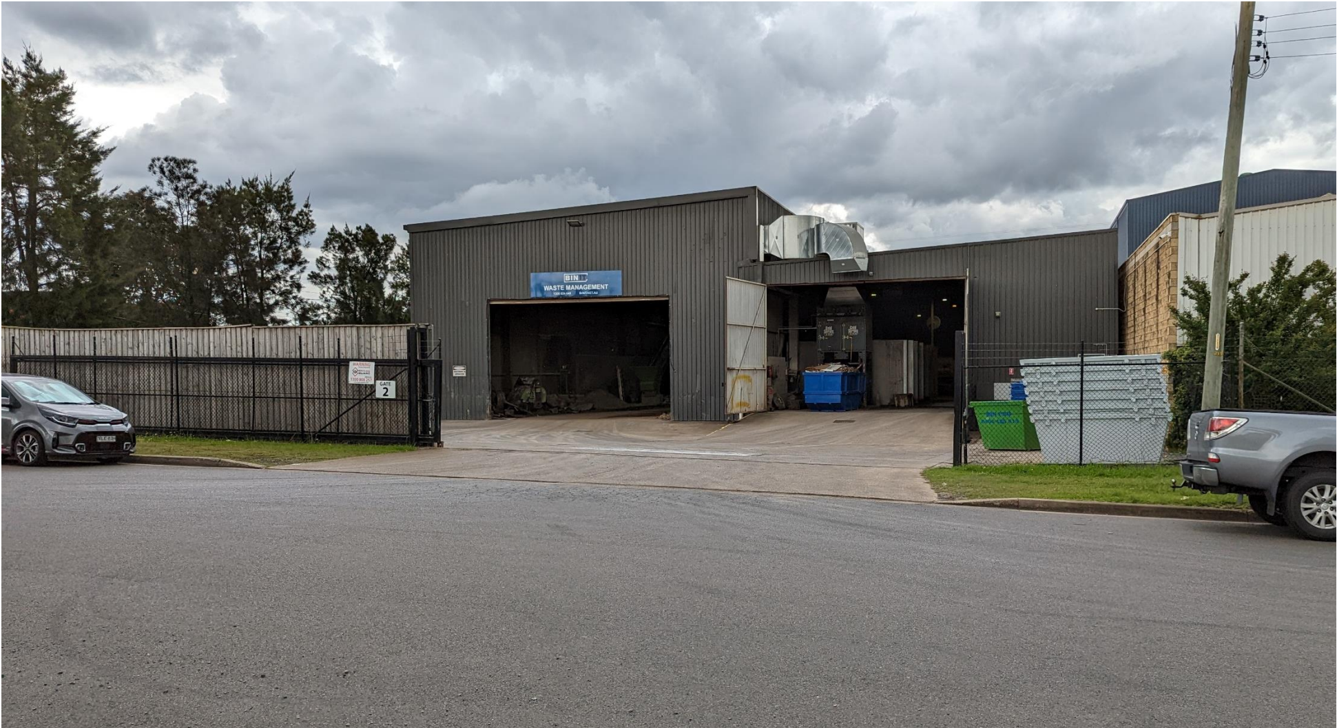
Figure 13.1. View of the front of 33-37 Plasser Crescent (Lot 16 DP 263353) showing dominant Site features.
